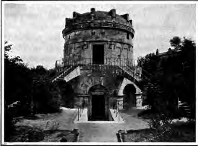
4. THE TOMB OF THEODORIC AT RAVENNA.—The most important Gothic monument in existence. The roof is hewn from a single huge rock and weighs nearly a million pounds.
